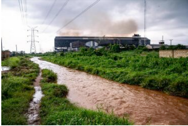
Rain water mixed with lead acid flows into Ipetoro community. Photos: Adetona Omokanya
